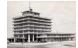
Tokyo Customs Headquarters Building completed in 1964
