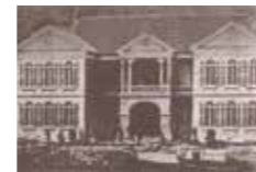
Kobe Customs Headquarters Building built in 1873
